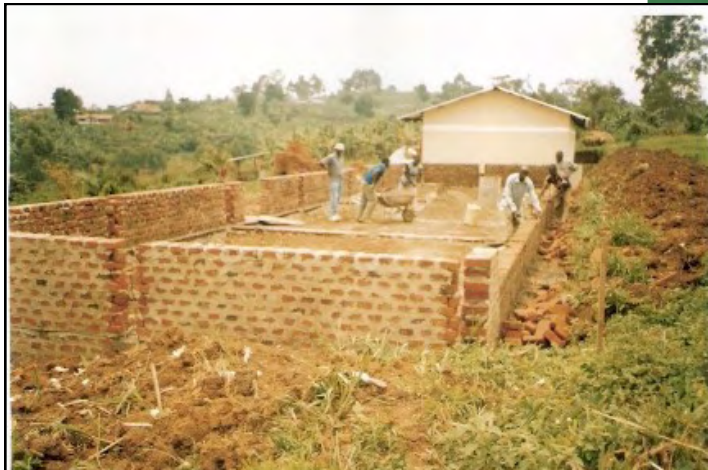
The construction process of the classrooms at Shalom Junior School as of September 2008.
